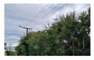
The **Growth Limit Zone** is the minimum clear space required to surround the electricity line in all directions as specified in the Regulations. The actual distance (in metres) is determined by the span length, conductor type and voltage of the electricity line.
