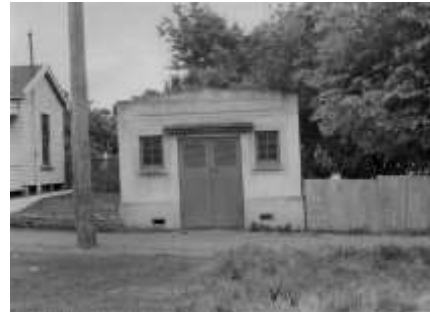
Bronte Street substation 1950 – still in use today
