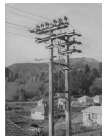
Stoke-Nelson transmission line 1954
