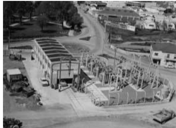
Electricity switchyard constructed 1959 finally decommissioned in 2013
