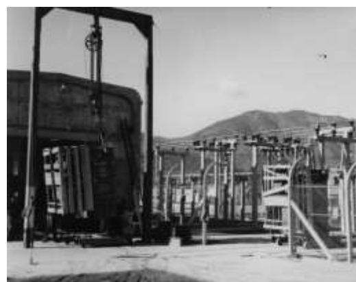
NEL's 33kV transformers arriving in Jan 1960
