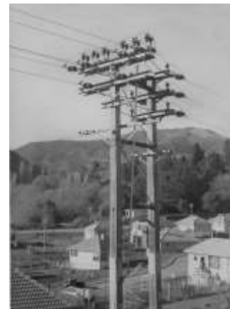
Stoke-Nelson transmission line 1954
