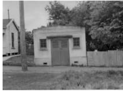
Bronte Street substation 1950 – still in use today
