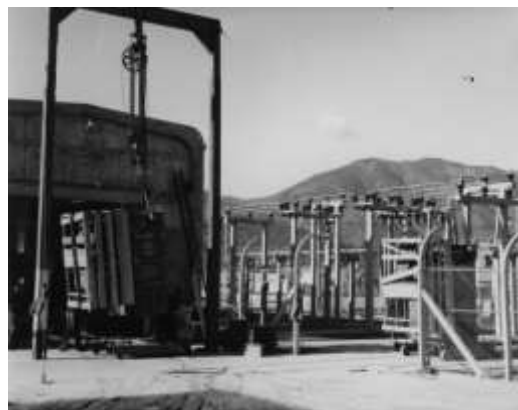
NEL's 33kV transformers arriving in Jan 1960
