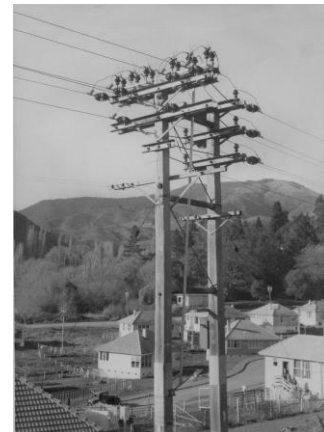
Stoke-Nelson transmission line 1954
