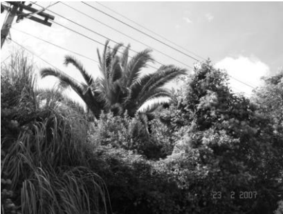
Trees close to powerlines Feb 2007
