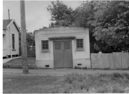
Bronte Street substation 1950 – still in use today
