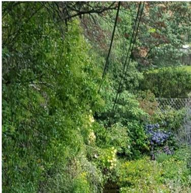
The **Growth Limit Zone** is the minimum clear space required to surround the electricity line in all directions as specified in the Regulations. The actual distance (in metres) is determined by the span length, conductor type and voltage of the electricity line.
